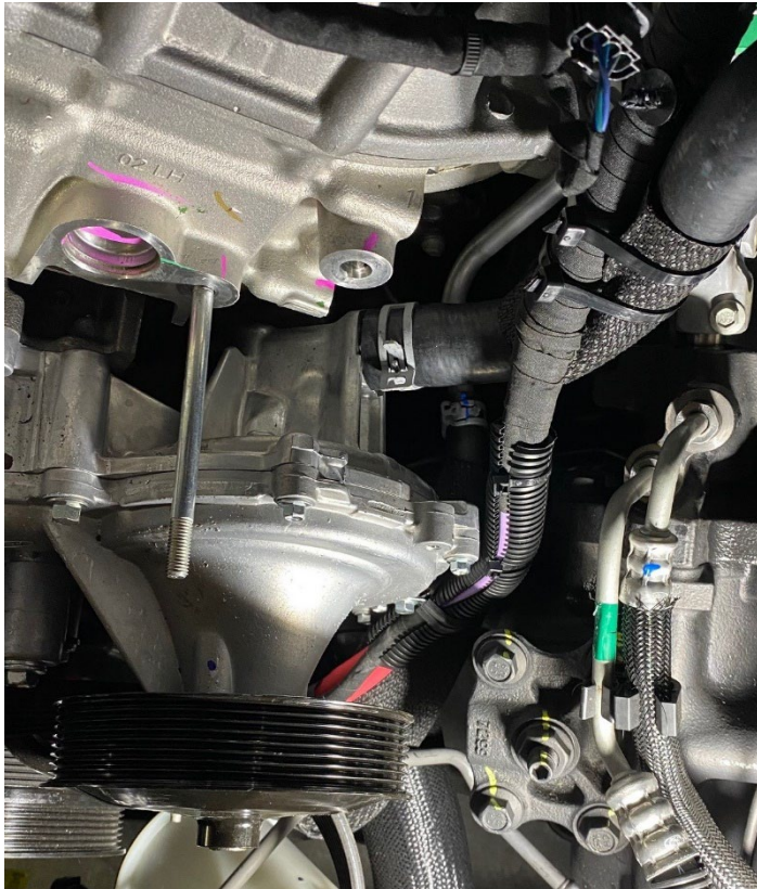
Battery Cable Support Hardware (17-21)
