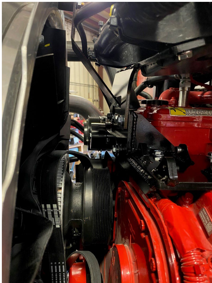
Fan Ring Support Bracket Installed
