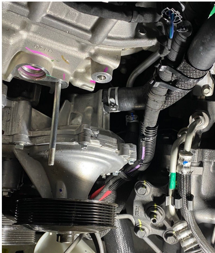
Battery Cable Support Hardware (20-24)
